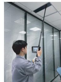
ceiling duct inspection
